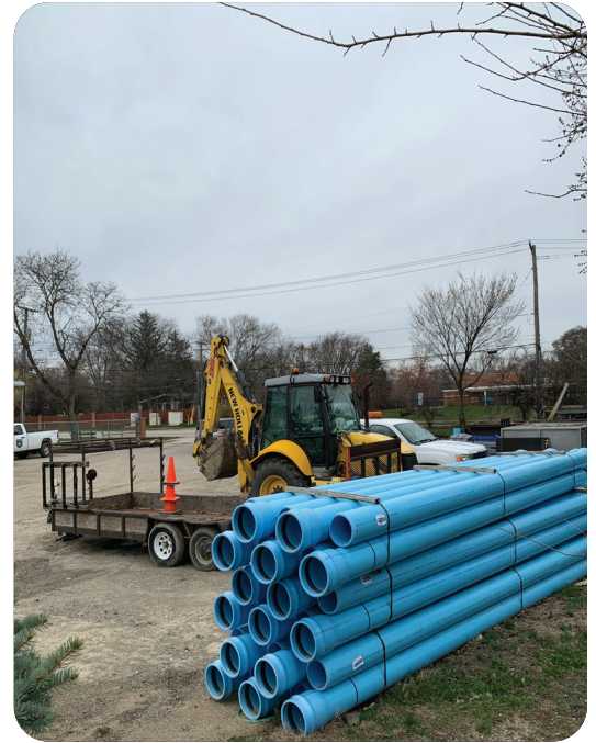
Lathrup Village DPS yard (Giffels Webster, 2020)
