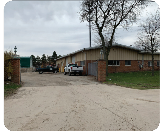
Lathrup Village DPS yard (Giffels Webster, 2020)
