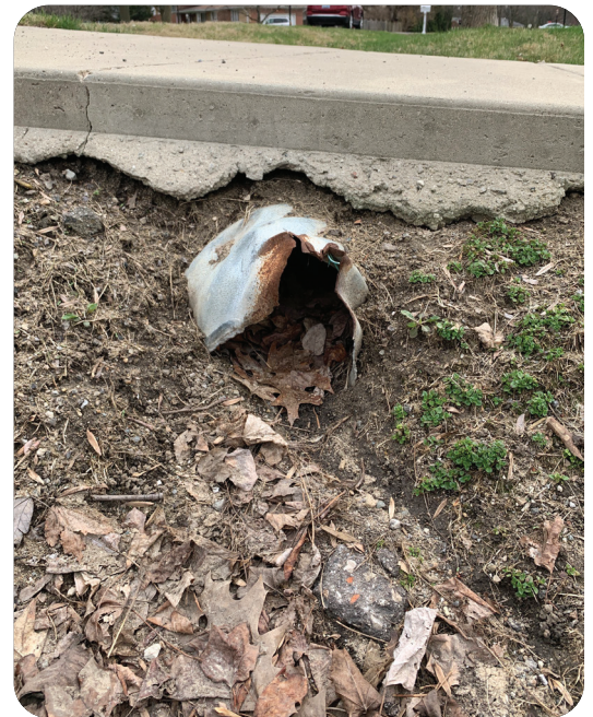
Damaged storm sewer culvert (Giffels Webster, 2020)
