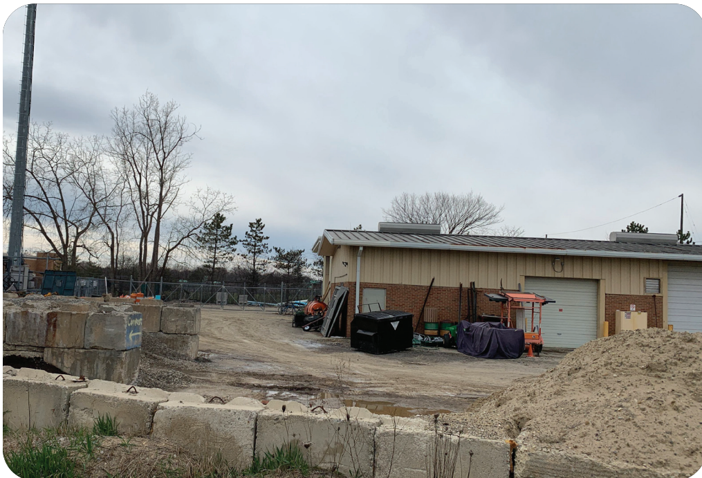
Lathrup Village DPS yard - entrance and front parking lot (Giffels Webster, 2020)
