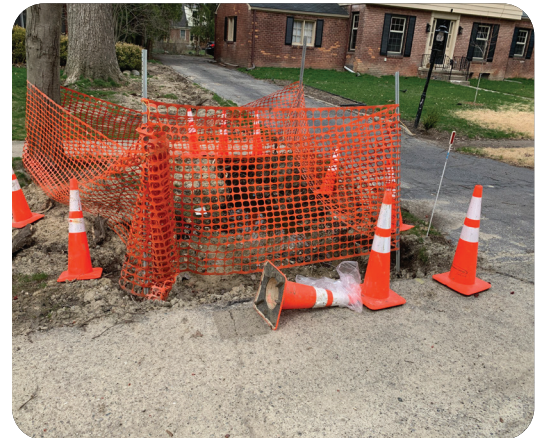
Drainage ditch repair (Giffels Webster, 2020)
