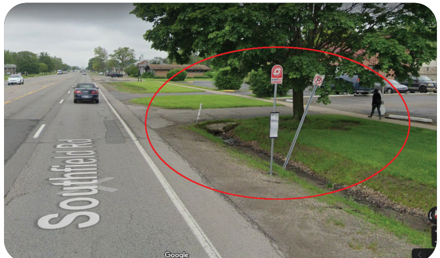
Existing bus stops on Southfield Road in need of safety upgrades (Giffels Webster, 2020)
